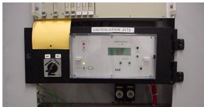
Fig. 1 – Frontal view of the controller installed in the utility substation.
