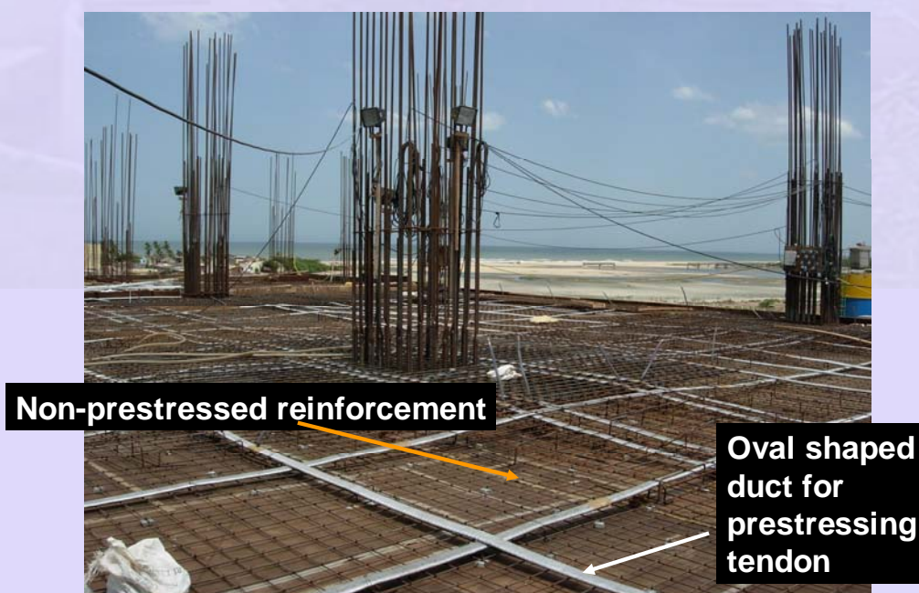
Figure 9-3.10 Reinforcement in a two-way slab (Courtesy: VSL India Pvt. Ltd.)
