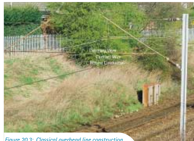
Figure 20.3: Classical overhead line construction
