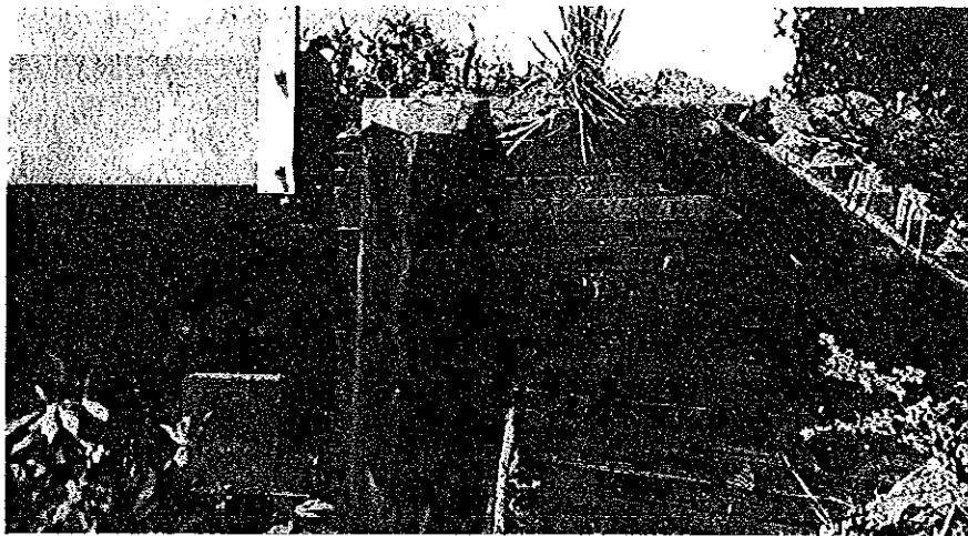
This laminated backwall and wings of pressure treated 2x4's was designed and built about 13 years ago by F. R. Rankin, county engineer of Reno County, Kansas.
