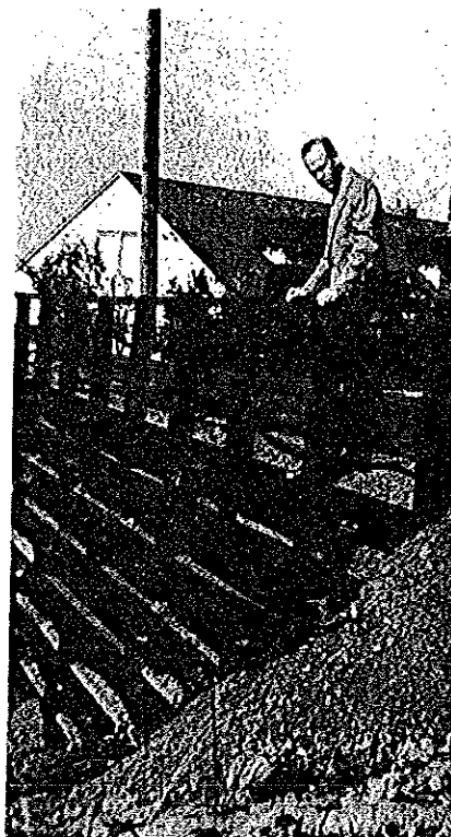
Pressure-treated crib-type retaining wall at residence in Portland, Oregon.
