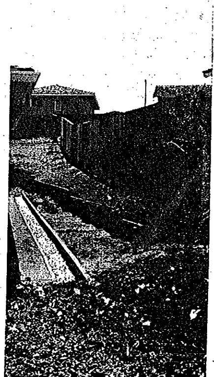
Typical of pressure-treated wood retaining walls found in residential areas, garden of residence in Menlo Park, California.
