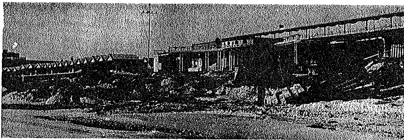
Collapse of inadequately designed seawall at Virginia Beach, Atlantic Coast, during March 1962 storm permitted tidal flow to
