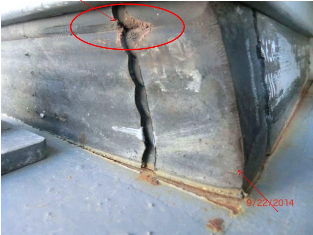
Photo 2, Bearing at G1 looking northeast; southwest corner rotated approximately 1/2 " east
