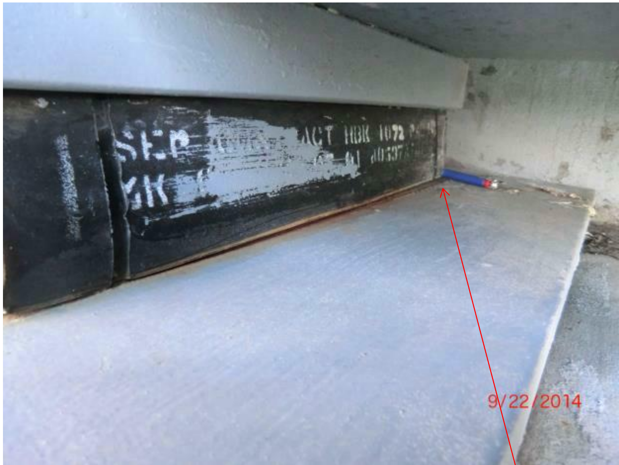
Photo 1 – Bearing at G1 looking northeast, southeast is rotated approximately \frac{1}{2}^{\circ} to the north
