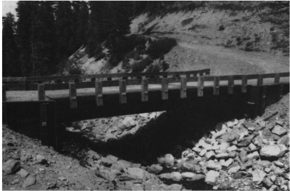
Figure 6-12. - A timber bridge with sharply curved approach roadways. Trucks crossing the bridge can produce centrifugal forces that affect the bridge superstructure and substructure.
