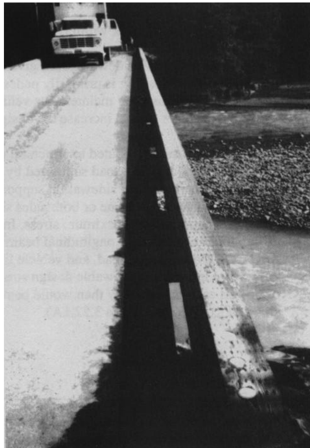
Figure 6-27—Barrier curbs on a timber bridge. Such curbs are sometimes used instead of railing on single-lane, low-volume bridges.
