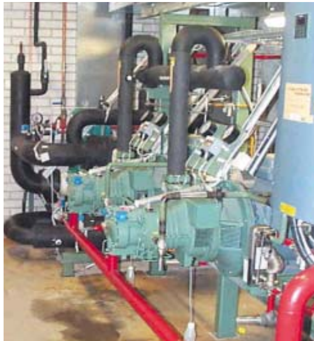
Figure 13. Two screw compressors.
