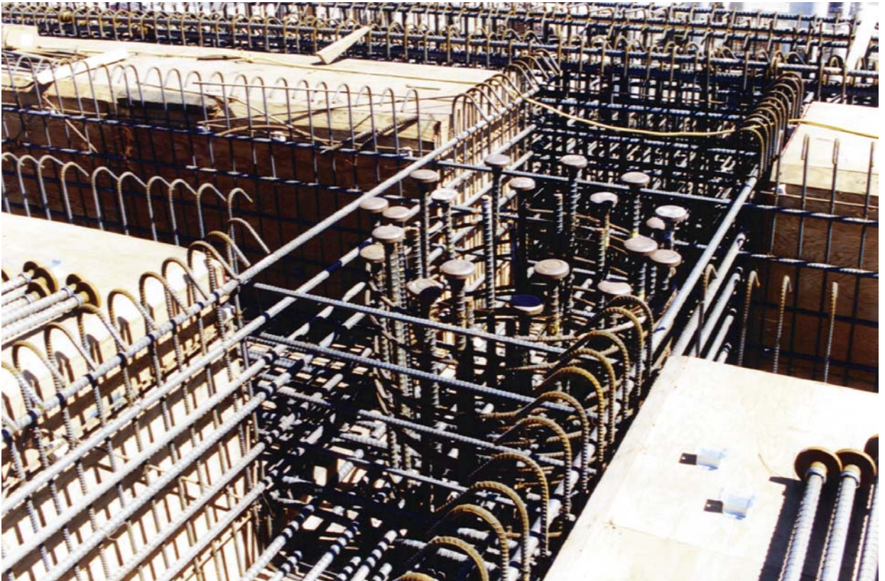
Figure 9 Headed reinforcing bars on the top of longitudinal column bars.
