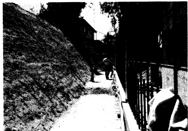
FIG. 9. Back-Cut Slope for Retaining Wall Construction
