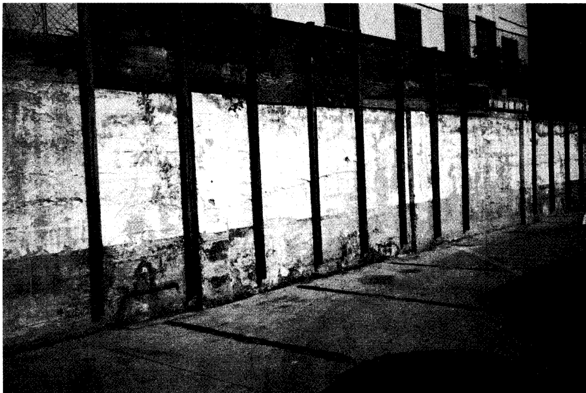
FIG. 1. Cantilevered Retaining Wall
