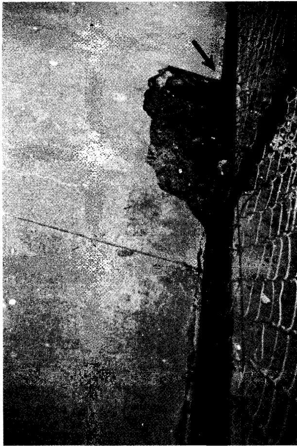
FIG. 4. Voids that Developed below Flatwork as Result of Wall Movement
