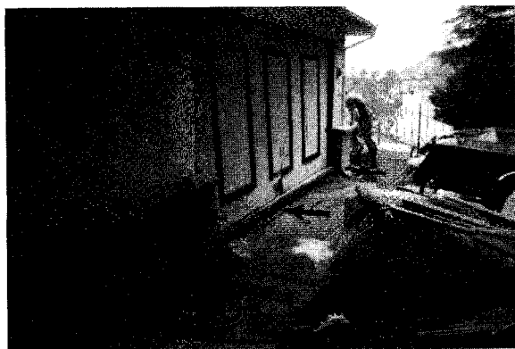
FIG. 7. Backfill Settlement as Result of Northridge Earthquake
