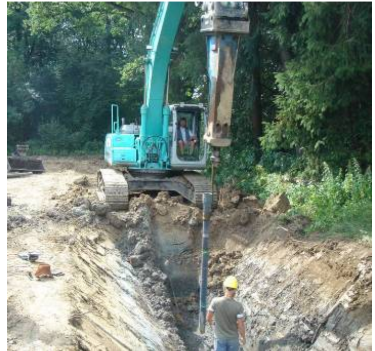
Pile-supported sewerage hydraulic network, Pennewang, Austria.
