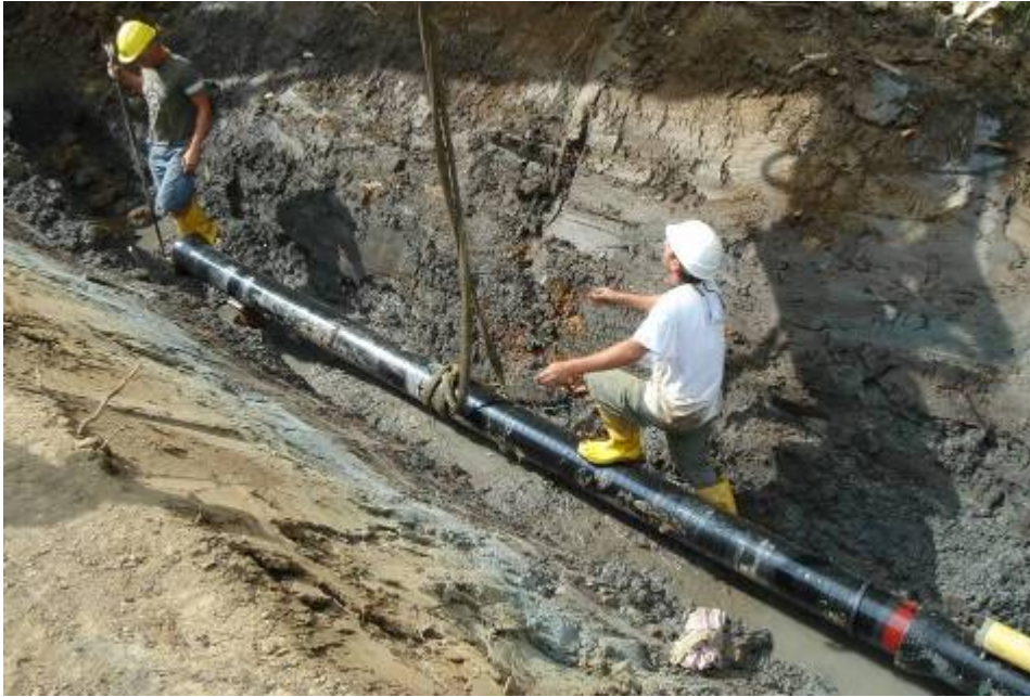
Pile-supported sewerage hydraulic network, Pennewang, Austria.
