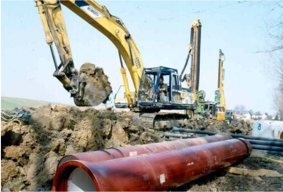
Pile-supported sewerage hydraulic network, Gunsirichen, Austria.
