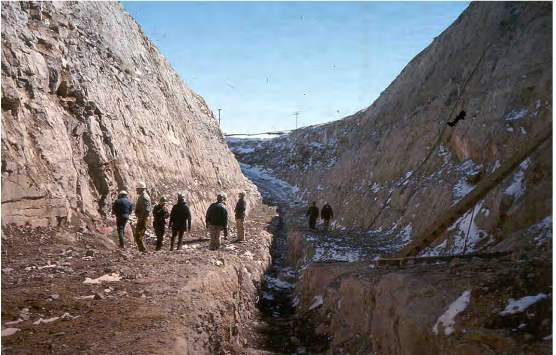
Fissure in D/S Right Abutment
