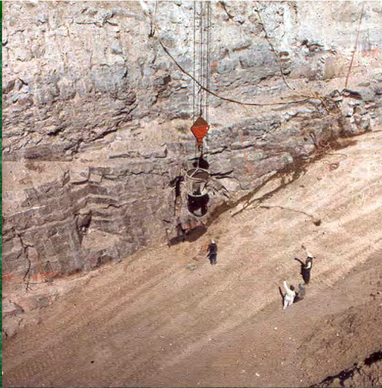
High Slump Concrete Placement
