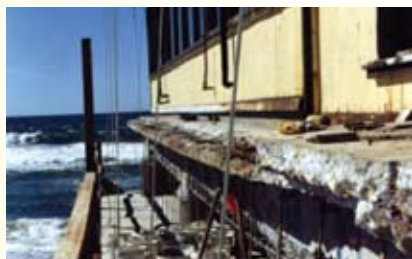
Figure 1 (left): Structure exhibits extensive corrosion caused by proximity to the ocean. Figure 2 (right): Repaired Structure. Along with extensive concrete repair, the fiberwrap system was designed to provide additional shear and flexural capacity.
