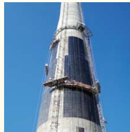
Figure 5: Fiberwrap being installed on a chimney. Work is performed by small crews from scaffolding.
