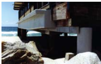
Figure 1 (left): Structure exhibits extensive corrosion caused by proximity to the ocean. Figure 2 (right): Repaired Structure. Along with extensive concrete repair, the fiberwrap system was designed to provide additional shear and flexural capacity.
