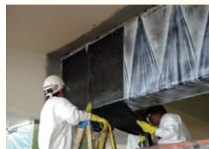
Figure 3: Carbon fiberwrap is installed over fiber anchors to provide confinement and shear capacity to beam end.
