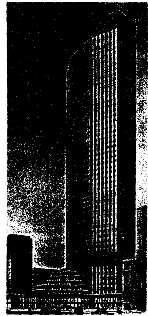
IDS CENTER, Minneapolis, Minn. 57 stories, towers over the Northwest. 1.4 million sq. ft. of Inryco 3"N and 3"NF deck. Owner: Investors Diversified Services, Inc., Minneapolis. Architects: Philip Johnson/ John Burgee, New York; Edward F. Baker Associates, Inc., Minneapolis. Structural Engineer: Severud, Perrone, Sturm, Conlin & Bandel, New York. Gen. Contractor: Turner Construction Co., Minneapolis.
