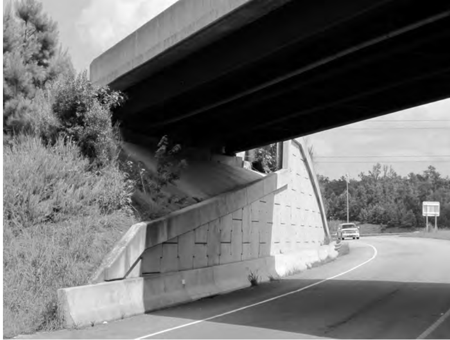
Figure 3.15.1-4. A steel girder bridge where a small mechanically stabilized earth (MSE) retaining wall was used to reduce the severity of skew without significant increase in span length.
