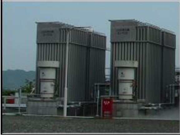
Figure 10. Ambient Air Vaporiser (Source: BV 2009)
