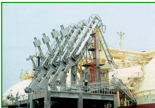
Figure 6. Unloading arms at an import (receiving) terminal (Source: BV 2009)
