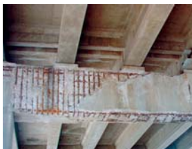
Figure 1 Spalling concrete under bridges signifies a deteriorating structure and presents a safety hazard for traffic below.
