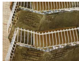
Figure 2 Black reinforcing bars are exposed by spalling concrete on the underside of these stairs. This unsightly deterioration is unsafe for people to use.
