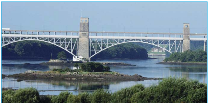
Britannia Bridge, Anglesey - 20mm Grip-Bar® used on strengthening internal bay anchor beams
