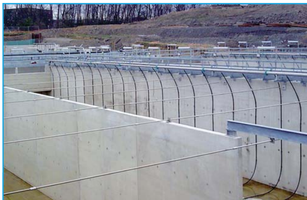
39mm Grip-Bar® tie bars at a Water Treatment Plant
