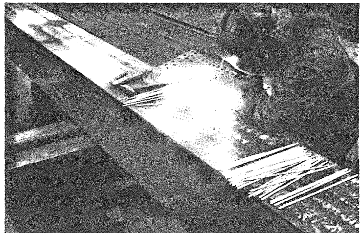
FIGURE 11C—The butt welded splice, easily made with downhand welding procedures, is entirely suitable for most driving conditions.
