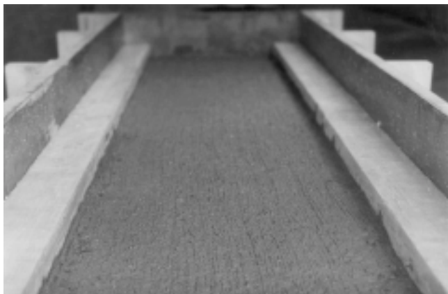
Fig. 12—Close-up view of broomed joint surface.
