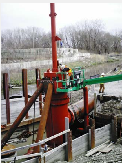
The 60-inch tap inserted a custom-made folding plug head that articulated to fit snugly inside the main line. With the bypass flow operating, the general contractor installing the rerouted line connected the new 90-inch water main. The system was then switched back over from the bypass line to the relocated 90" line without incident.
