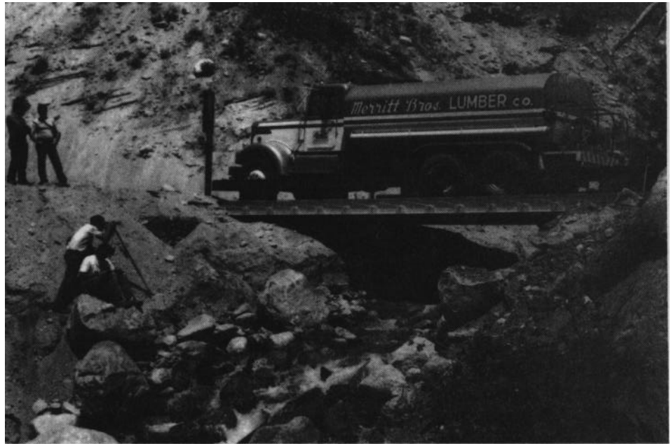
Figure 9-5. - Load test of the Zuni Creek stress-laminated deck on the Idaho Panhandle National Forests.
