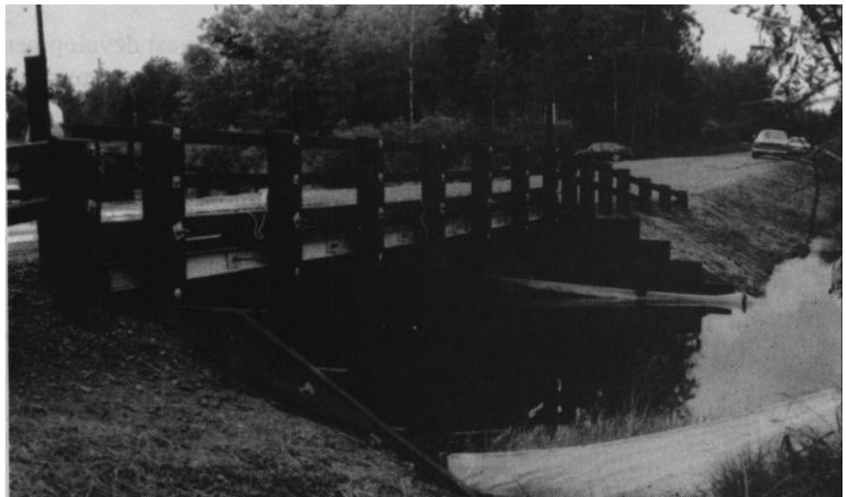
Figure 9-2. - Stress-laminated deck bridge built over Iron River on the Chequamegon National Forest in 1988.
