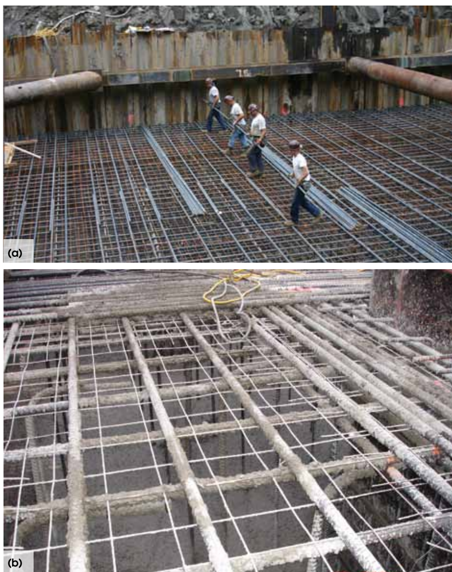
Fig. 7: WWR placed between the top reinforcing bar layers allows the workers to safely walk on the mat before and during concrete placement: (a) Trump Tower, Chicago, IL; and (b) Roosevelt University, Chicago, IL (photos courtesy of Jack Gibbons, CRSI)
