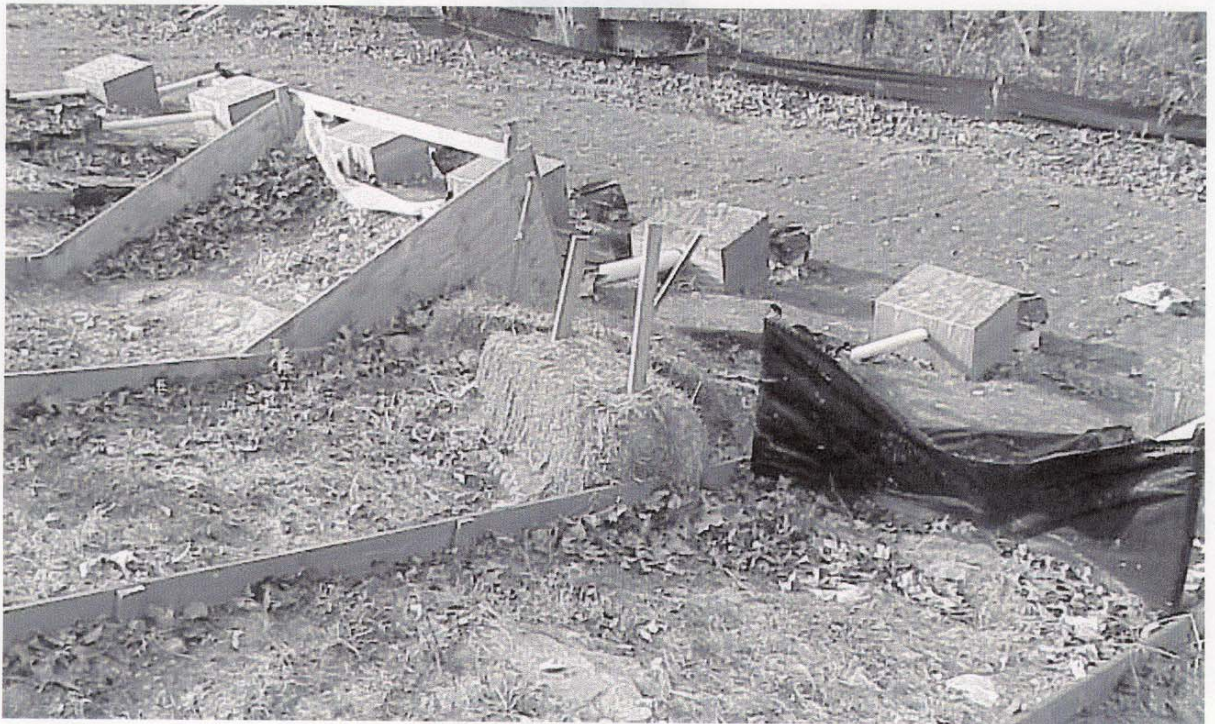
Figure A-2 View of Filter Berm, Hay Bale and Silt Fence
