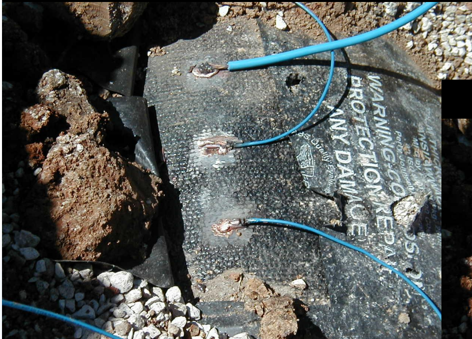
Raw Connections before Coating
