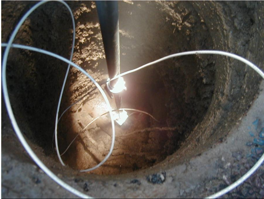
Exothermic Welding Tool Down the Hole
