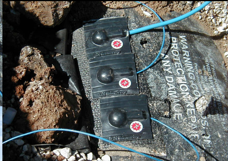
Finished Connections Ready to Backfill
