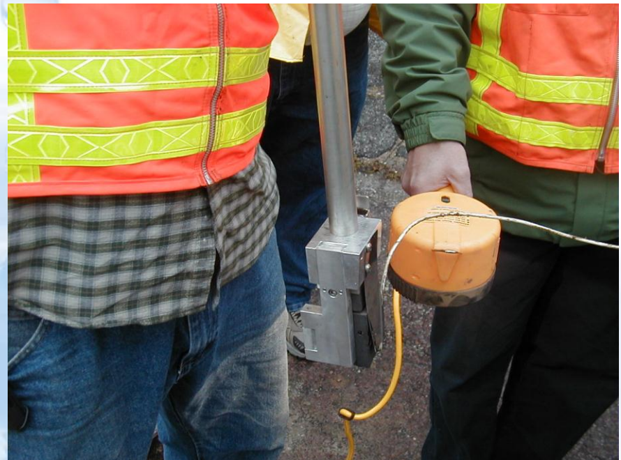
Anode Lead Wire into Welding Tool
