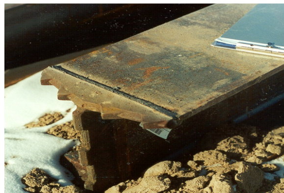
Figure 3. Pile drive point attachment.
