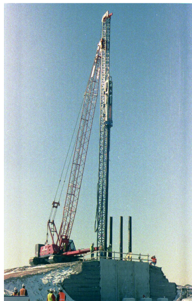
Figure 1. Pile diving through a full-height precast concrete panel faced geogrid-reinforced MSE wall.
