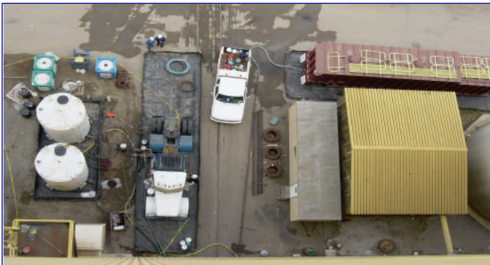
Typical Turbine Foam Job Chemical Mix & Waste Storage Layout
