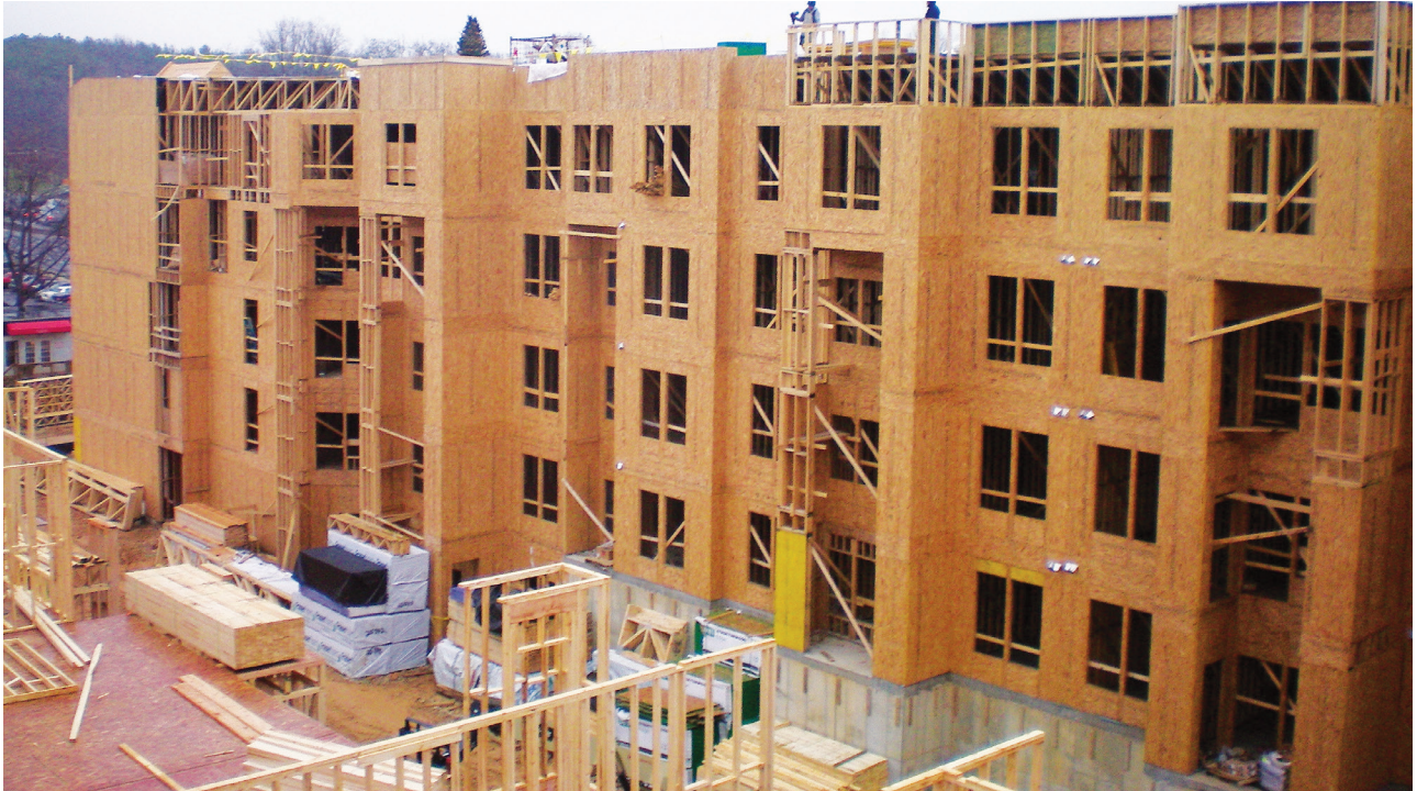
When structural panels such as plywood or oriented strand board (OSB) are properly attached to lumber floor, roof and wall framing, they form diaphragms and shear walls that are exceptional at resisting seismic forces.
