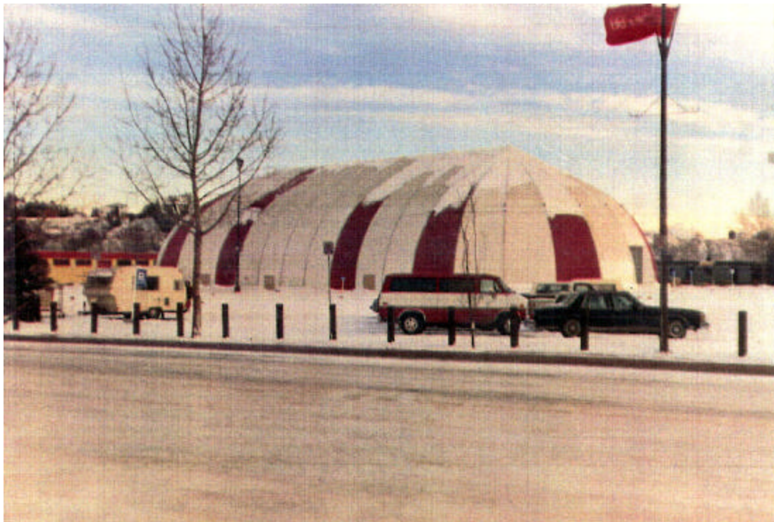
Calgary, Alberta Ground Snow Load 19 psf Picture taken one day after 4" snowfall Note: Evidence of snow sliding from roof (Photographs C-9 and C-10)
