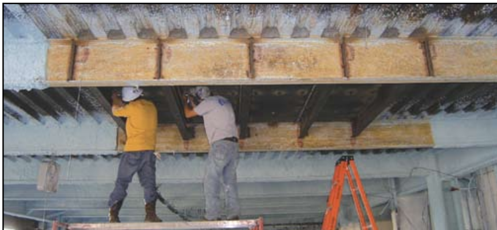
Figure 8: Structural repairs to limit floor slab displacements.
