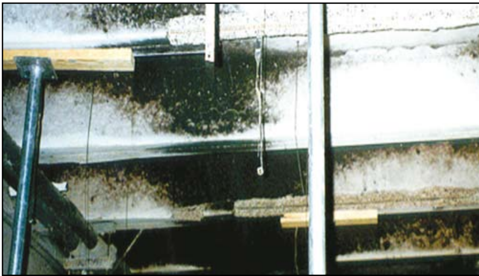
Figure 2: Slab separation and joist spalling.
