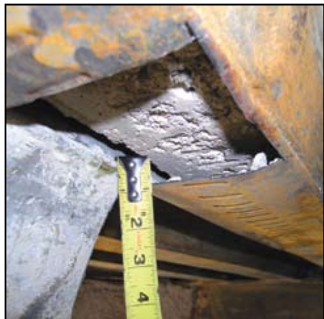
Figure 6: Buckled metal deck. Note separation of concrete from metal deck through exploratory opening.
