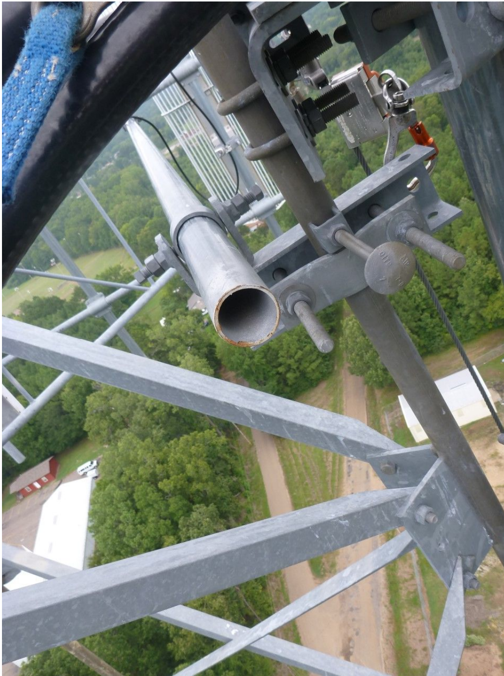
Figure 1: Antenna Mount Tieback Connection Picture
