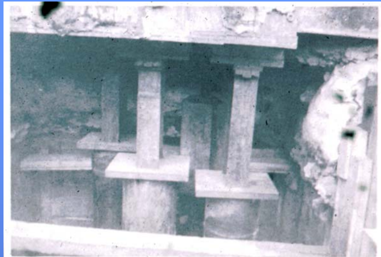
PILE GROUP READY FOR CONCRETING
