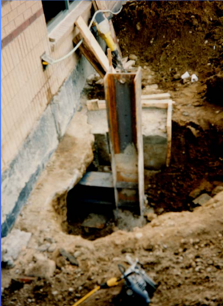
Bracket pile installation
