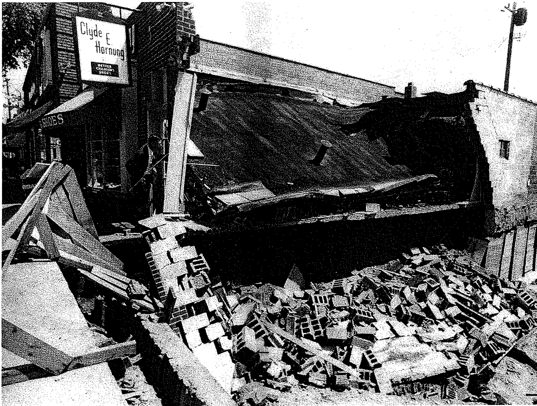
Fig. 22.5 Collapse of small building due to improper underpinning and lateral support.
