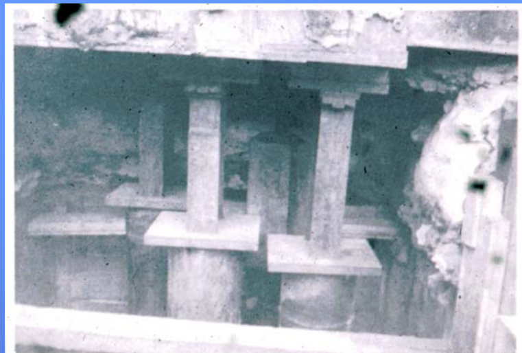
PILE GROUP READY FOR CONCRETING
