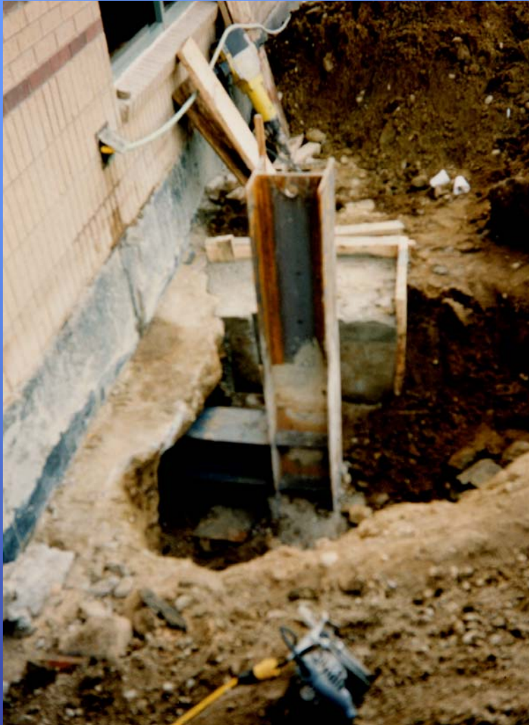
Bracket pile installation
