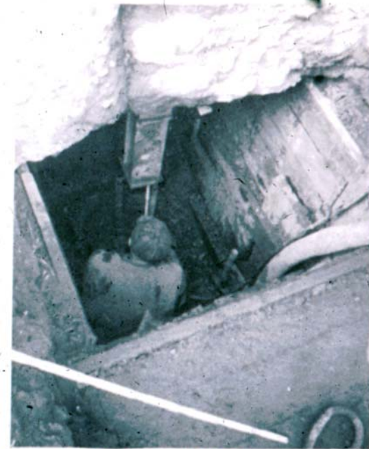
MEASURING MOVEMENT OF INDIVIDUAL PILE
