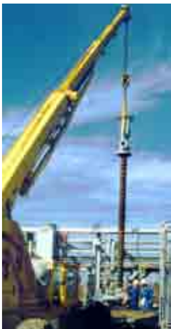
Figure 10. Pump Assembly Being Removed.
