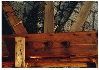
Two other factors contributing to timber truss failures involve the connections between the individual truss members. Truss joint design developments in the 1930s resulted in the use of multiple split-ring or bolted fasteners that inadvertently create semi-rigid
