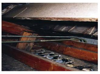
indicative of potentially damaging roof leaks. Evidence of deterioration at truss ends may include dark discoloration of the wood, crushing of the curved top chord member end against the steel shoe, elongation of bolt holes, splitting of chord members, visible reverse curvature of the top chord and visible, localized sagging of the bottom chord (see Figure 6).
