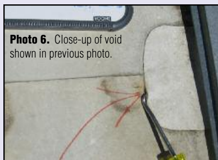
Photo 7. Depicts a small void in the weld of a flashing collar flange at Roof Area 1 of the Seattle, Washington site. Note that flashing collars are hand-welded.
