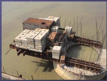
Kentledge being used to correct for tilt in sinking
