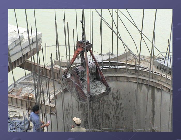
Digging out soil to sink well foundation
