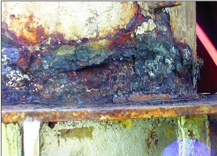
*Effects of corrosion under insulation near angles on steel*
