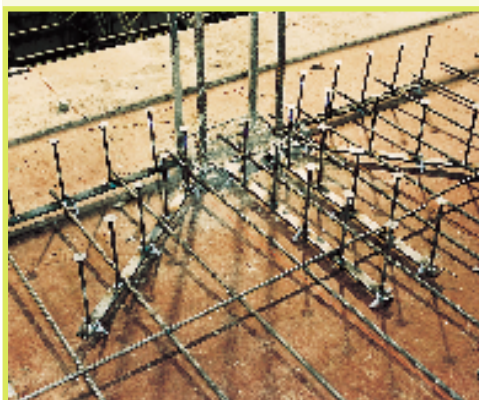
Figure 2: Stud rails arranged radially around an edge column
