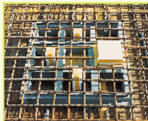
Figure 6: Structural steel shearhead allows the formation of openings immediately adjacent to an internal column
