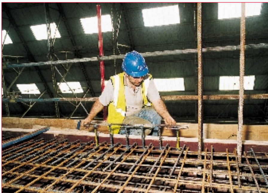
Figure 1: Fixing prefabricated shear reinforcement at Cardington
