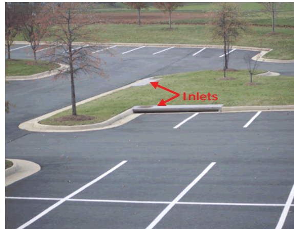
Two Curb-Opening Inlets at Low Spots
