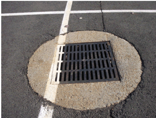
Figure 5 – A Grate Inlet
