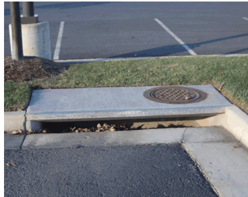
Figure 6 – A Curb-Opening Inlet
