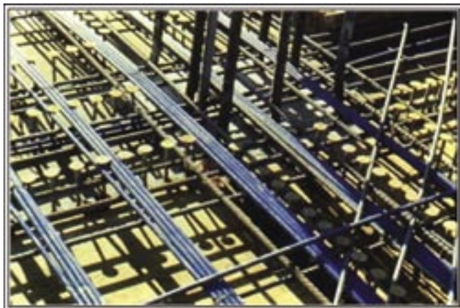
Fig. 2: This type of shear reinforcement is easy to install, without congestion or formwork interruption 5
