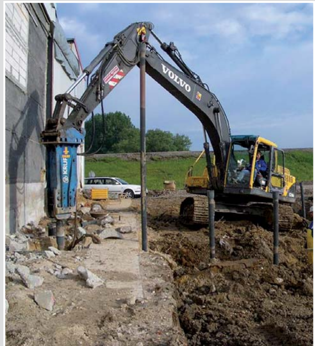
Foundation works adjacent to an existing building
