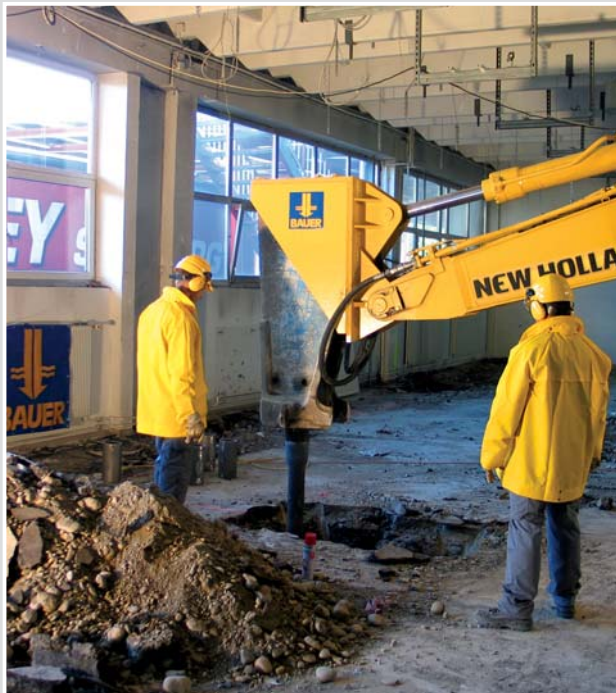
Underpinning works in restricted headroom
