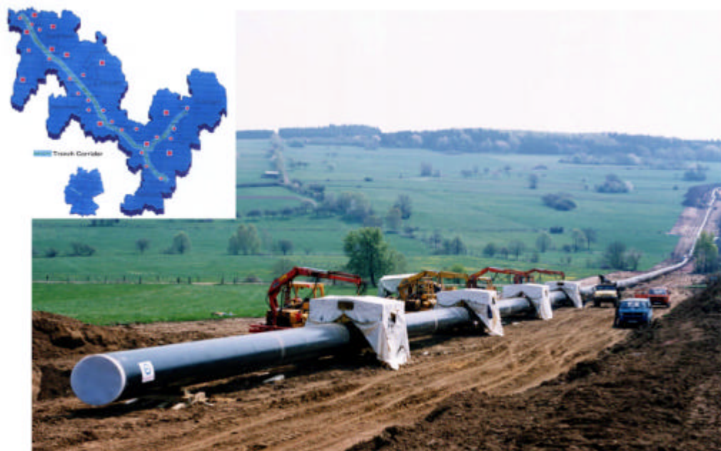
Figure 4: First large scale use of GRS 550 TM (X80) Pipe Line Material Ruhrgas Werne-to-Schlüchtern Line
