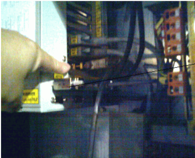
Rear view of an HFE (HFT) control box showing the HFE (HFT) cable connection
