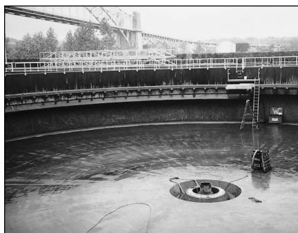
This photograph shows a secondary clarifier retrofit at a municipal wastewater treatment plant.
