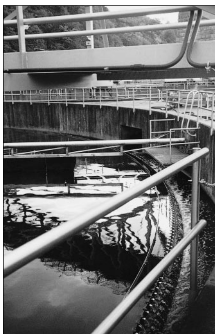
This is a close up of the weirs of the clarifier and shows the use of 316 stainless steel bolting.
