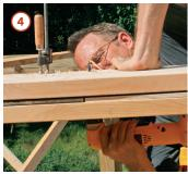
The steel is shorter than the rafters. Fill in the ends of the steel plate with 3/8-in. plywood and 1-in. roofing nails. After the top rafter is bolted in place, 8d nails driven from each side will hold the tails together.
