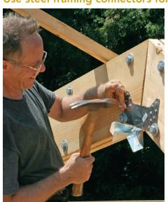
The steel flitch-beam assembly shoulders the shear load in one direction, but the intersecting hip rafters should be supported with a special framing anchor (the
