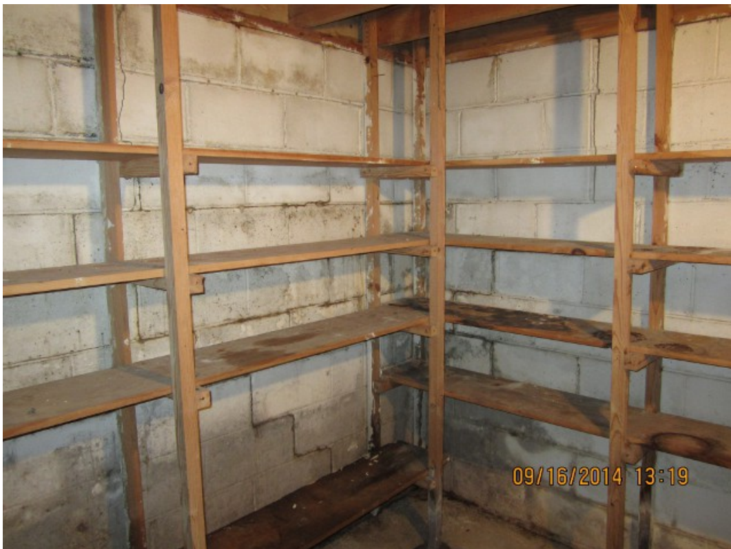
different bad corner. lots of cracking and out-of-plane movement
