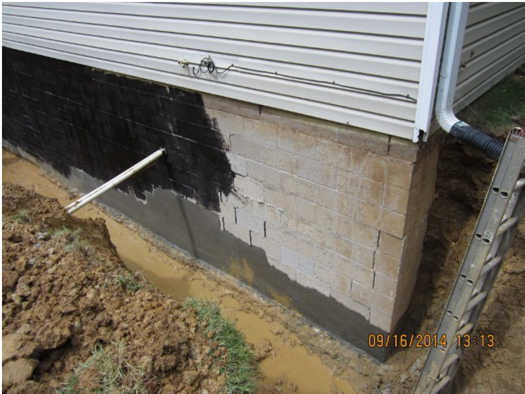
bad corner - vertical cracks at corner, and wall going to the left has moved inward at the top
