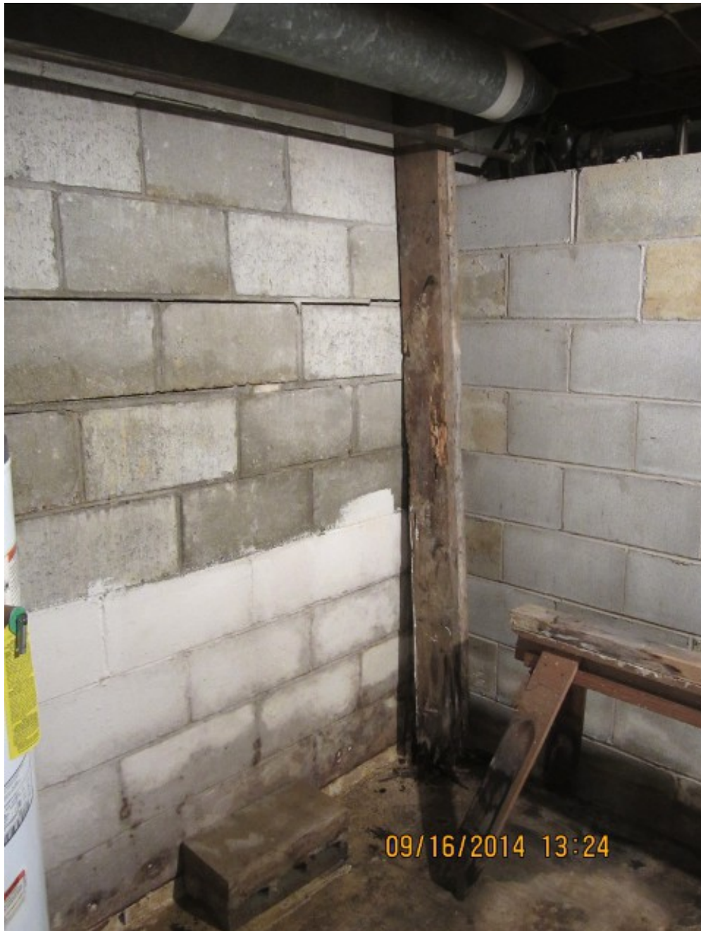
another bad spot. back wall with 4" deflection. CMU buttress and original wood "repair" - sheared off from rot
