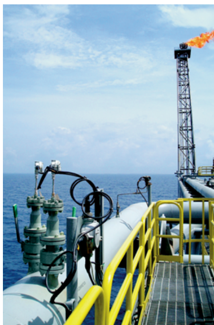
Figure 4: Isolating valves allow the transducers to be changed while the flare header is in service.
