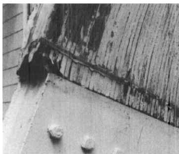
Figure 4-6. (C) Outward displacement evidenced by shear at the arch base.
