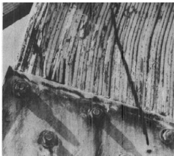
Figure 4-6. (B) Outward displacement evidenced by bend in laminations.
