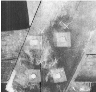
Figure 3-2. (B) No significant splits exist in the connector areas. The split shown is in the tension chord and does not pass through a connector. "X" marks were used as a "check off" for a previous inspection.
