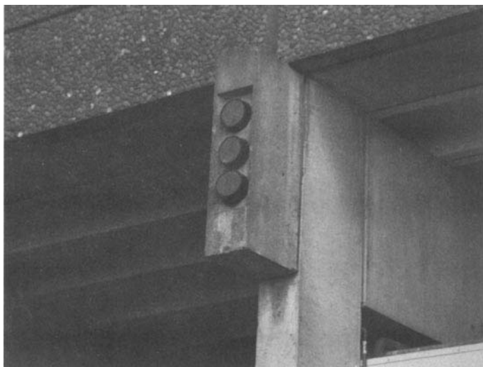
Expression of prestressing anchorage in a frame of the Students Association Building, University of Canterbury.
